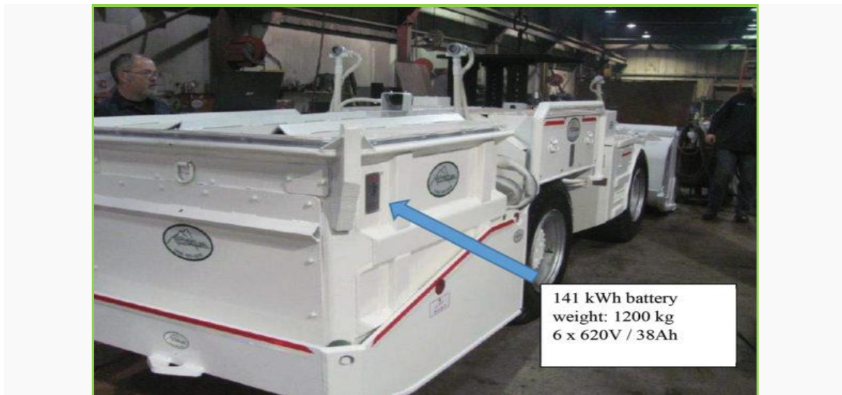
Figure 19 Sodium nickel chloride battery mounted on an LHD (Saminco).
