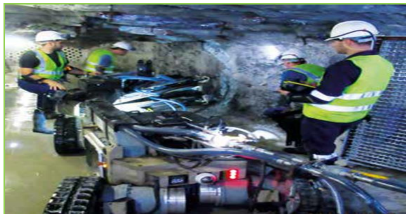
Figure 32 MT1000 Multi-drill during initial commissioning and sub-system testing (Sibanye Stillwater, 2018)
