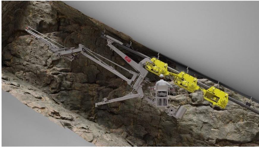
Figure 28 HPE narrow tunnel drilling rig on monorail (HPE, 2019)
