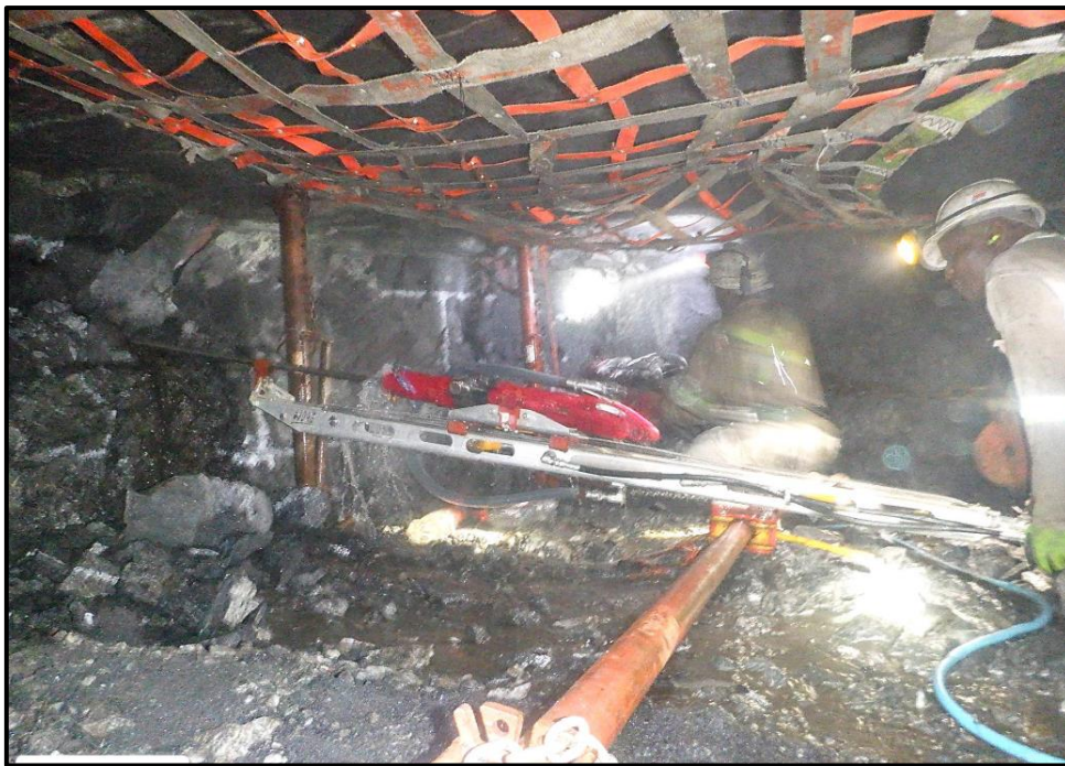
Figure 4: HPE Isidingo rock drill operating on a drill guide
