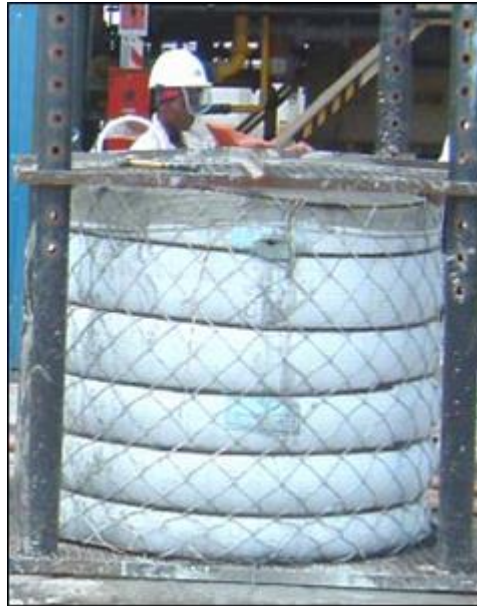
Figure 8. RSS grout pack constructed in a frame on surface (Grave, 2006)
