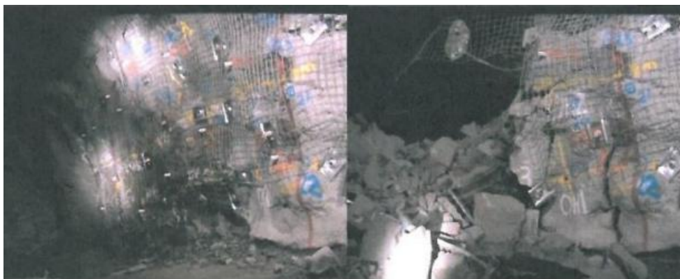
Figure 4: Before and after blast image captured by high-speed camera showing the damage to the tested support system (Heal & Potvin, 2007).
