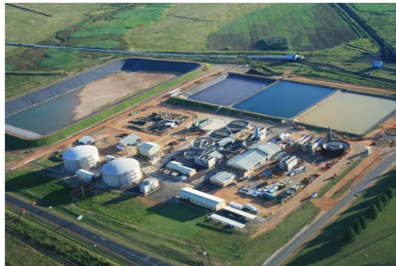
Figure 9: eMalahleni Water Reclamation Plant
