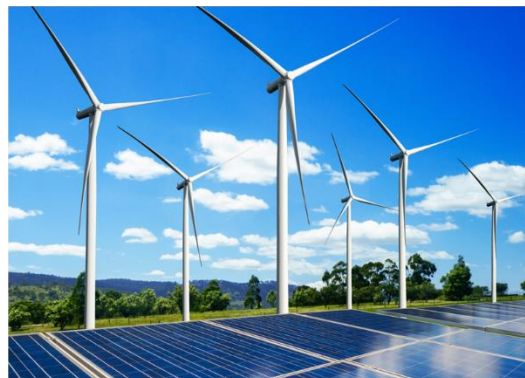
Figure 33: Solar PV and Wind System for Pilanesburg Platinum Mine
