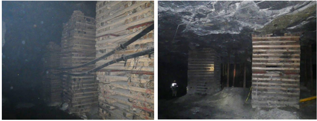
Figure 46. Castle packs in the area where the pillars were extracted.
