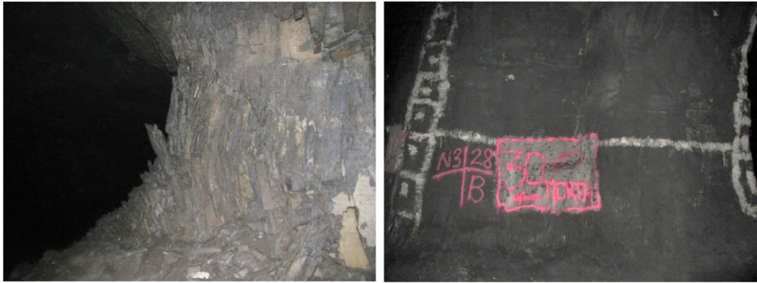
Figure 44. Different manganese pillar behaviour, in the same mine, caused by the number of joint sets and the spacing of the joints (after Wessels and Malan, 2023).
