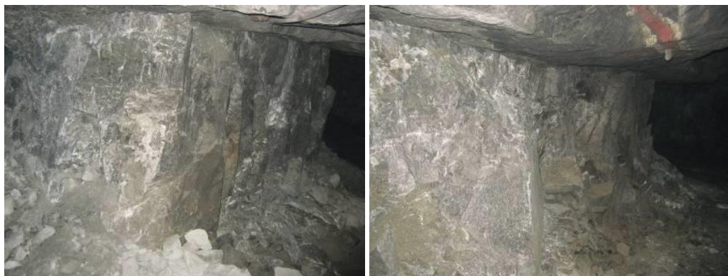
Figure 20. View of the sidewalls of pillar F
