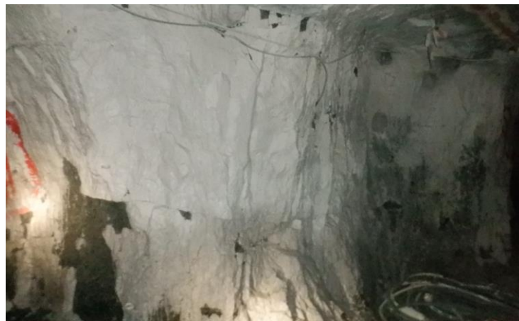
Figure 82. General condition of the pillars in the area visited. This is for pillar S74 DD P81
