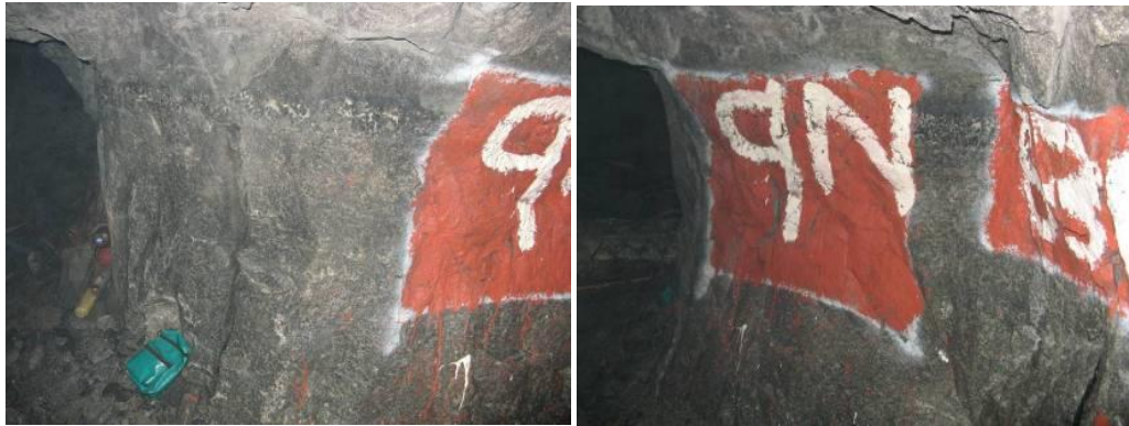
Figure 22. Examples of pillars adjacent to the face. Very little spalling was seen on these pillars
