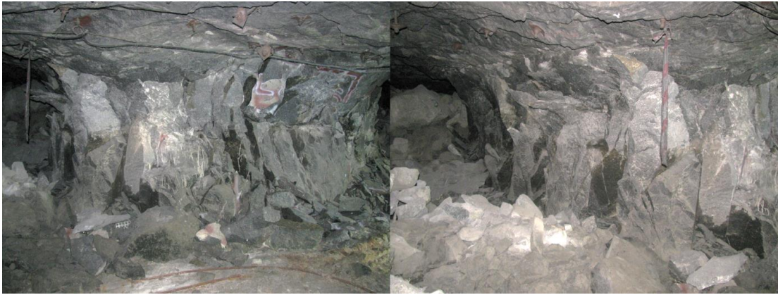
Figure 59. Photographs showing the observed conditions for S3W147
