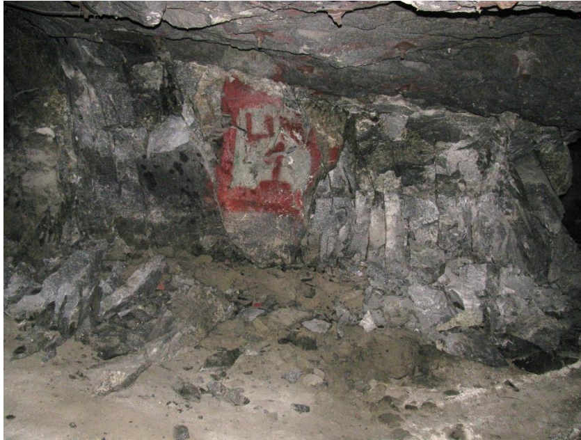
Figure 66. Typical high density of jointing in the recent area visit in the S3E and S3W areas
