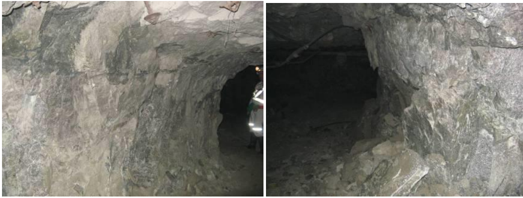
Figure 16. View of the sidewalls of pillar D
