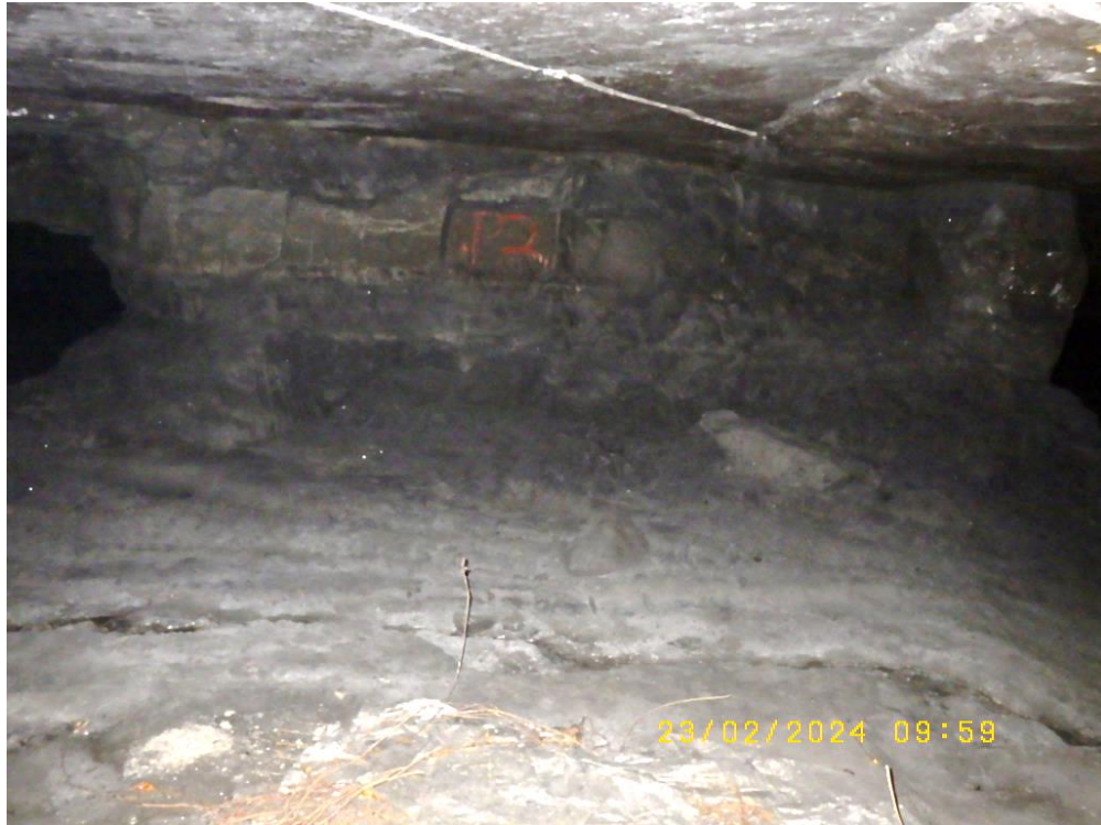
Figure 76. View of pillar 82. This pillar was still in a very good condition
