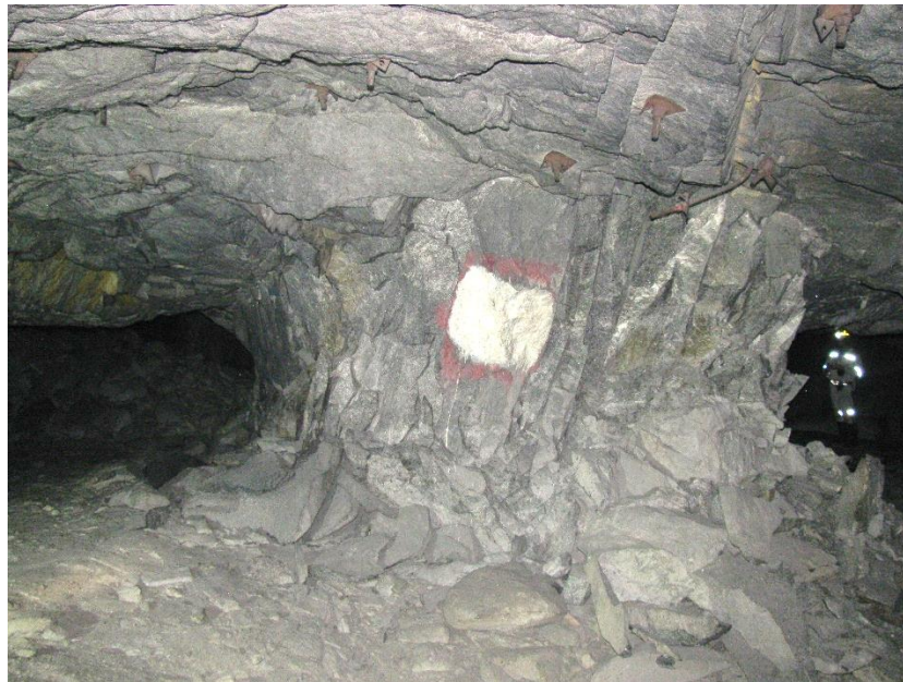
Figure 67. Another photograph of the high density of jointing in the recent area visit in the S3E and S3W areas. Note the continuation of the joints into the hangingwall
