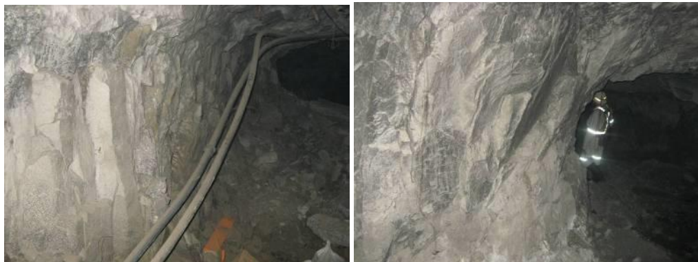
Figure 18. View of the sidewalls of pillar E
