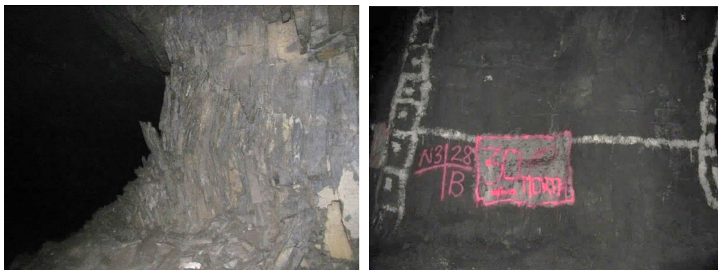
Figure 87. Differences in the behaviour of manganese pillars caused by the number of joint sets and the spacing of the joints (after Wessels and Malan, 2023)
