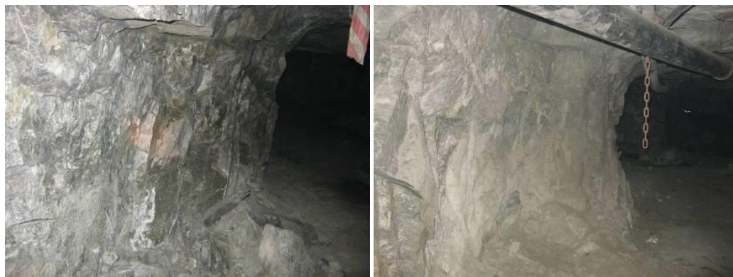
Figure 17. View of the sidewalls of pillar D
