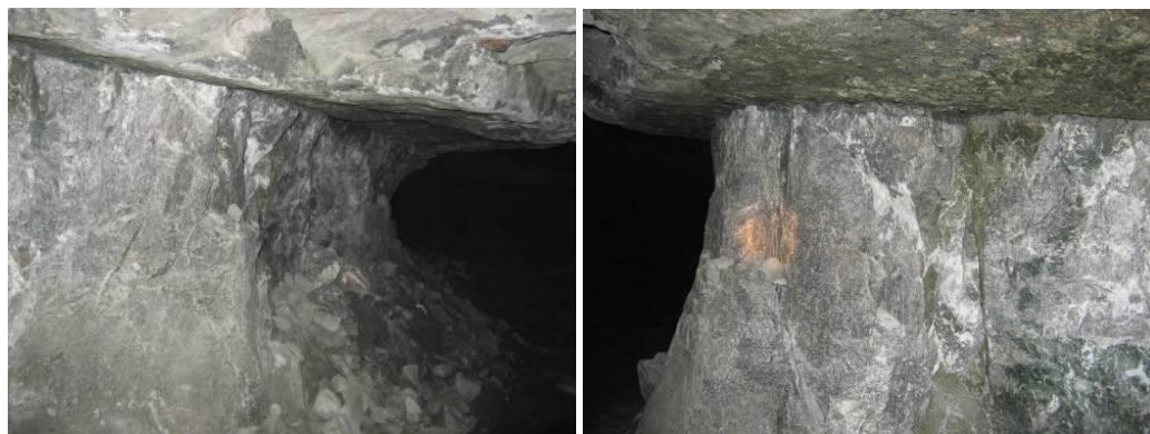
Figure 21. View of a sidewalls of pillar F. One of the corners is shown on the right
