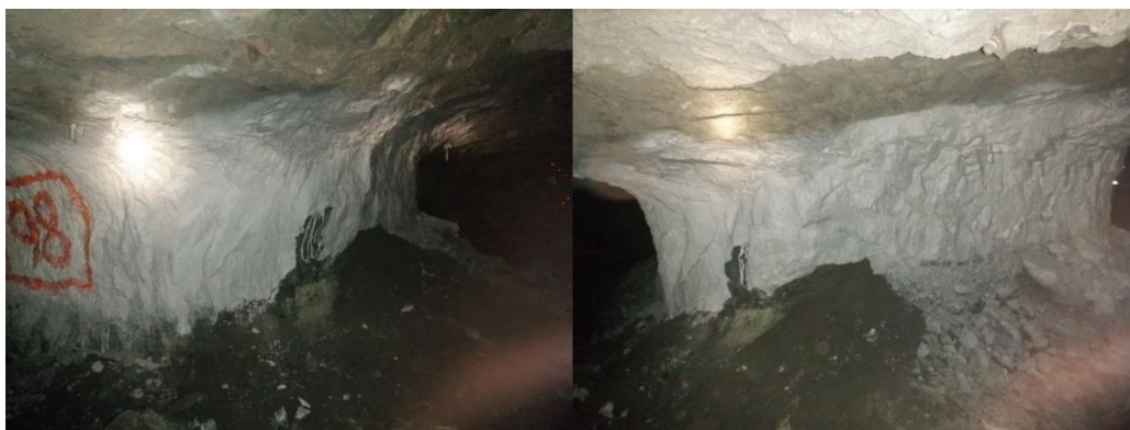
Figure 83. Photographs showing the condition of pillar S74 DD P98
