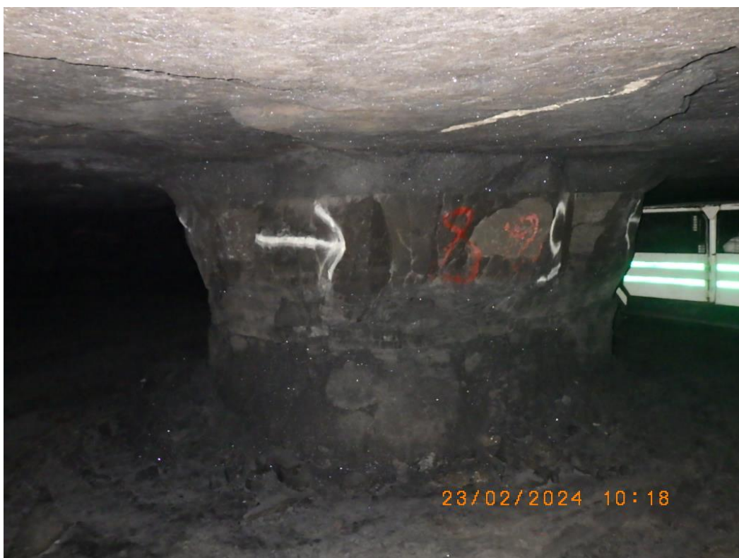
Figure 75. View of pillar 105. This pillar was still in a very good condition
