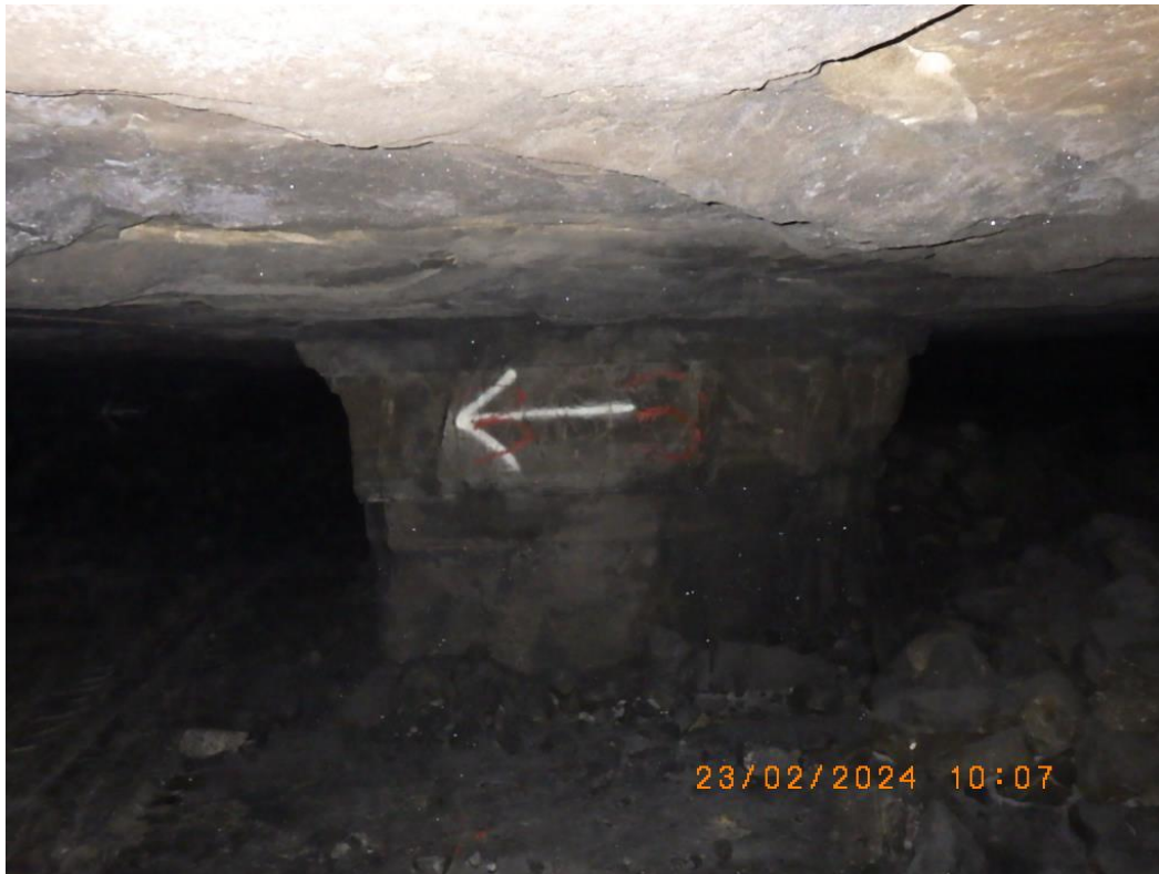
Figure 74. A photograph of pillar 93. This pillar was still in a very good condition
