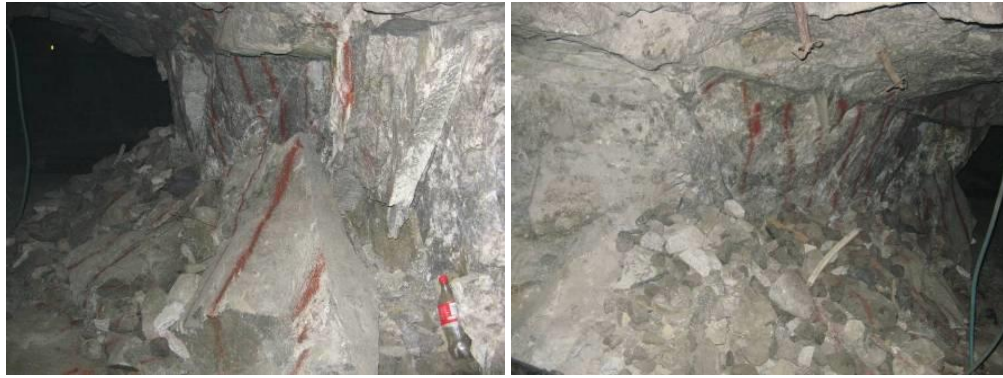
Figure 10. Spalling on the edge of pillar A
