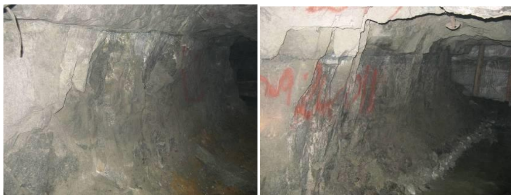
Figure 15. View of the sidewalls of pillar C
