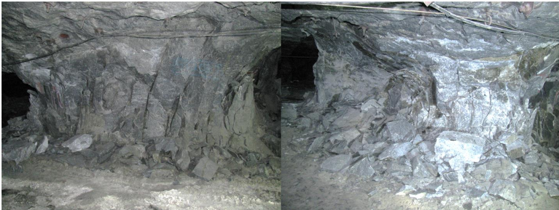
Figure 60. Photographs showing the observed conditions for S3W146
