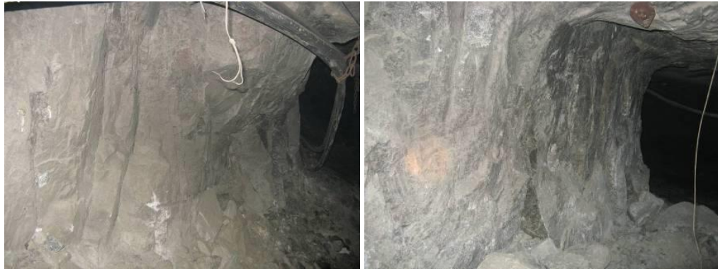
Figure 19. View of the sidewalls of pillar E
