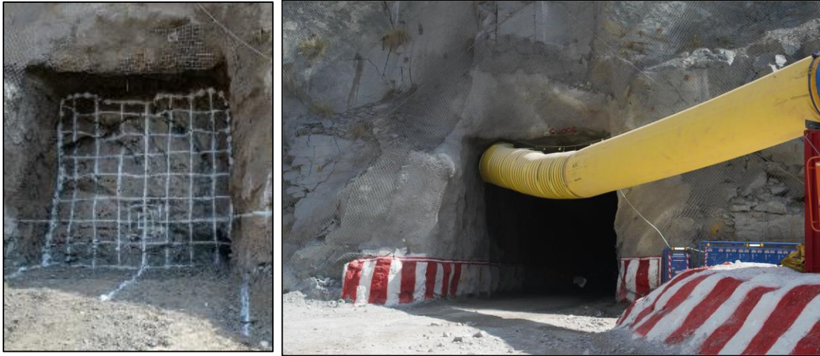
Figure 50. Images of the portal and post-development of the conventional drill and blast heading (Van Rooyen and Carstens, 2022)
