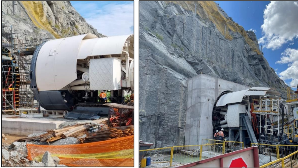
Figure 48. Images of the set-up of the MTB at Mogalakwena Mine (Van Rooyen and Carstens, 2022)
