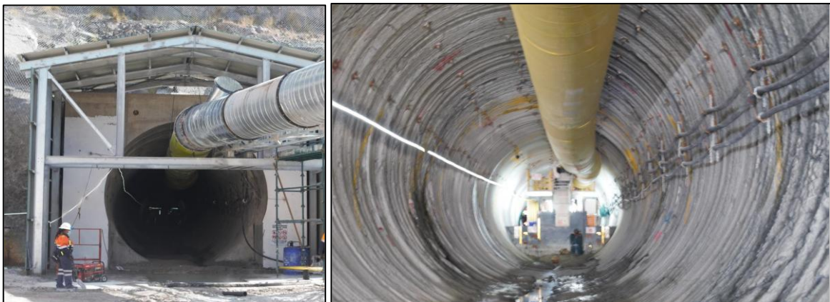
Figure 49. Images of the portal and post development of the MTB heading (Van Rooyen and Carstens, 2022)
